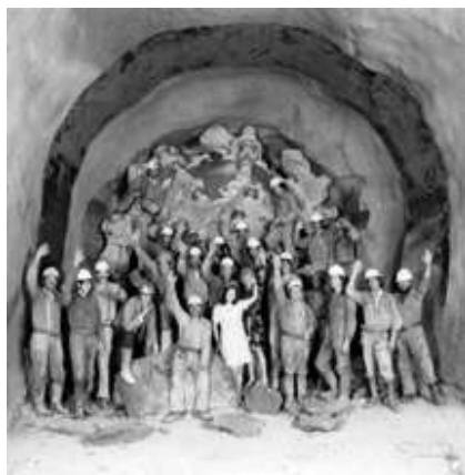
Proton Super synchrotron tunnel, 1974
