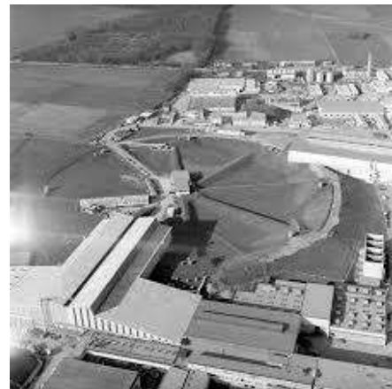
Cut and cover tunnel of the Proton synchrotron, 1959
