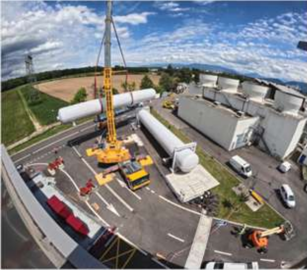
Two large helium tanks for the High-Luminosity LHC were installed at Point 1 in June. (Image: CERN)
