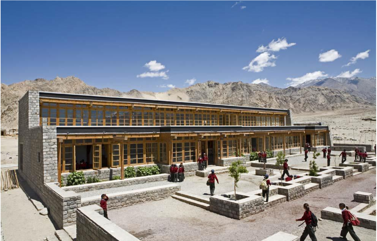
Druk White Lotus School in Shey uses building orientation and glazing to provide passive energy and maximize the solar potential in the high-altitude climate
