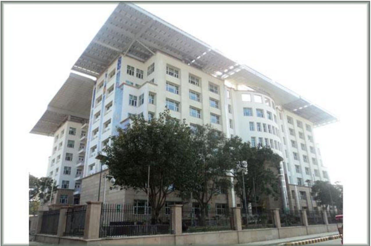
Indira Paryavaran Bhavan (IPB) in Delhi uses a combination of building design techniques to reduce the need for traditional air conditioning, including passive cooling, a chilled beam system for active cooling, and building materials designed for insulation and heat reflection
